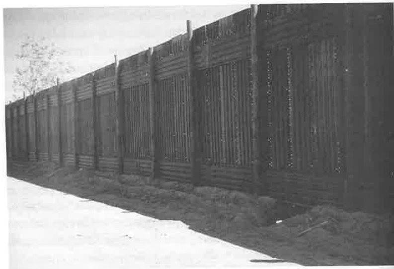
Figure 1. The new border fence made of corrugated iron landing mats recycled from an earlier war. Photograph by Armando Rascón.
